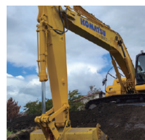
Slope Building in Pond
