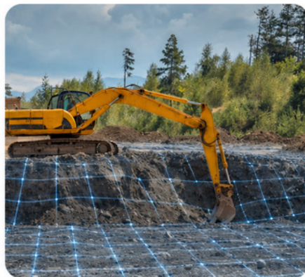
Slope & Embankment Construction
