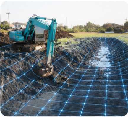
Farmland Drainage & Channel Construction
