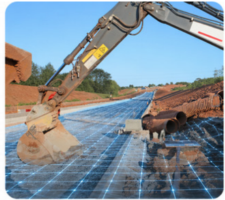
Roadbed & Subgrade Construction
