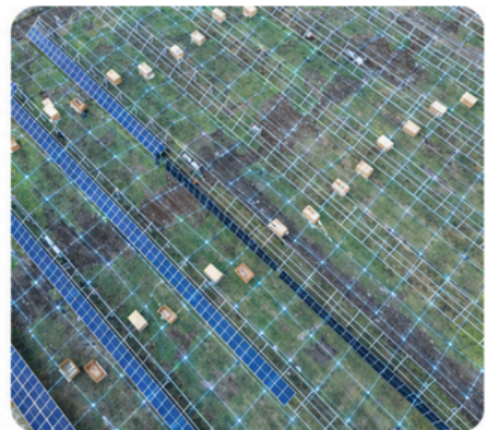
Solar PV Pile Layout & Installation
