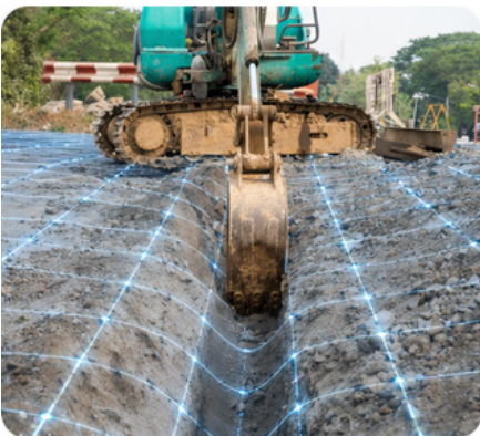
Road Alignment & Drainage Works
